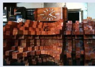
❶ The diffuser on the back wall of Florian Meindl's Berlin studio. "This is my self-constructed quadratic residue diffuser made of 284 wood parts," he says, "it diffuses the frequencies bouncing back behind me."
